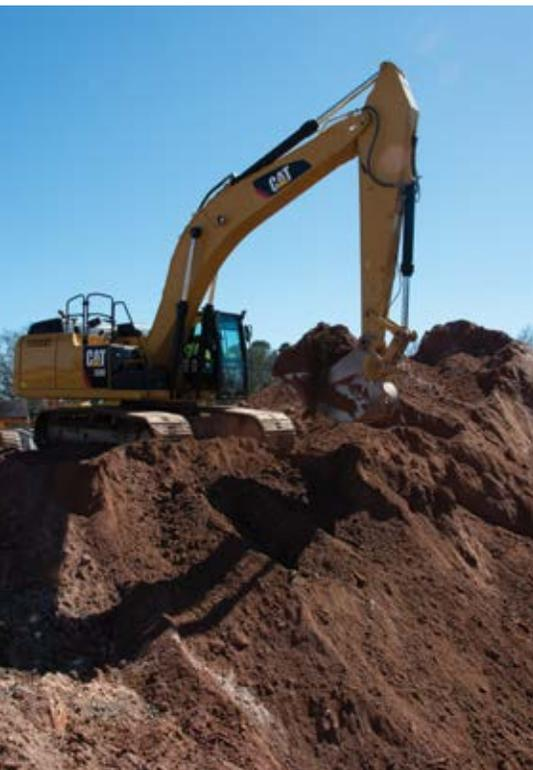
On one side of the jobsite, parking is being built on top of the underground detention pond. Centerpoint excavated about 15,000 cubic yards of dirt to install it and then backfilled it with 2,000 tons of #57 gravel stone and dirt fill the rest of the way up.
