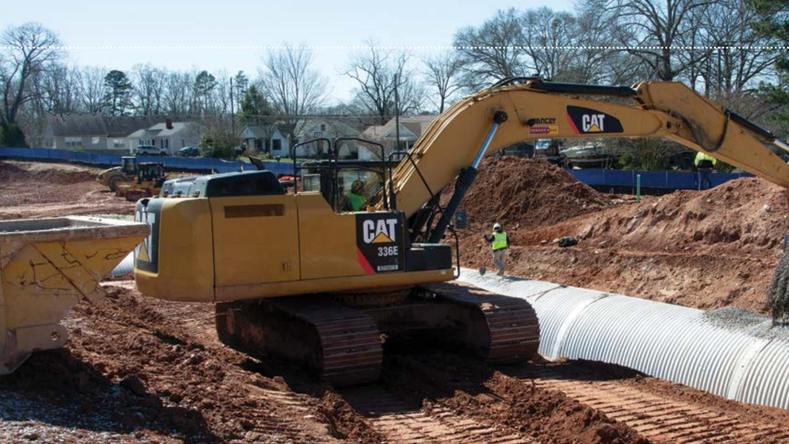
roughly 50,000 cubic yards of dirt, installing a 144-inch underground detention system approximately 600 feet in length, plus several other utilities that
